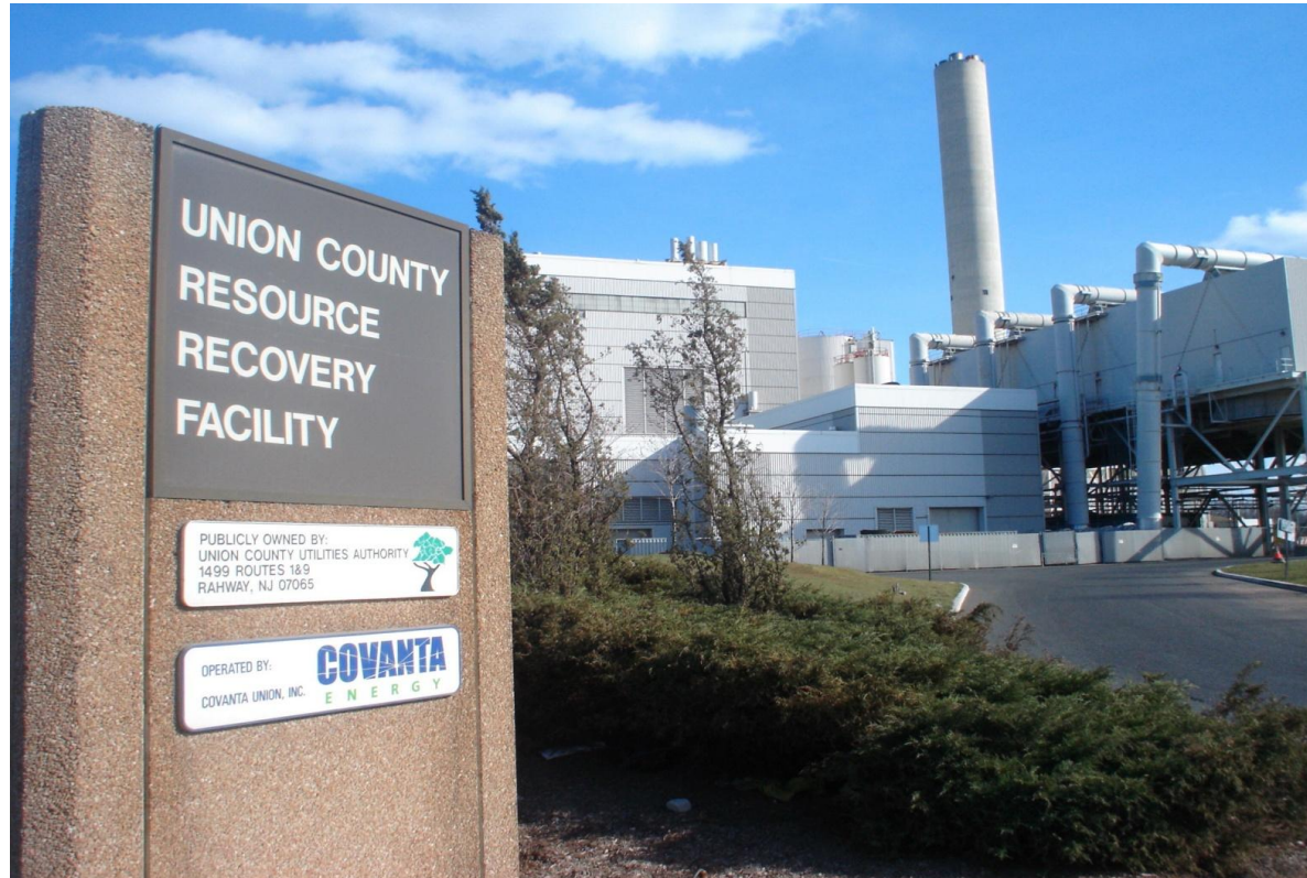
UNION COUNTY RESOURCE RECOVERY FACILITY
